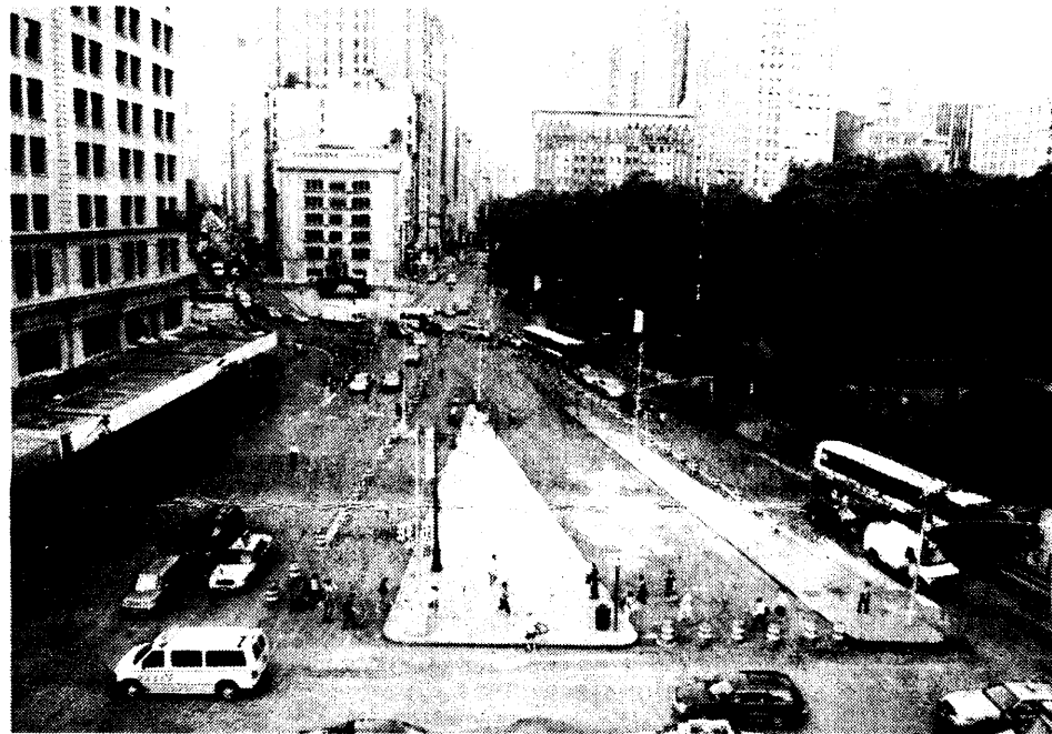
The area west of Madison Square Park, shown in a DOT photo taken last month, will soon become part of a pedestrian plaza.
